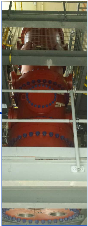
PFBC Pressure Vessel
